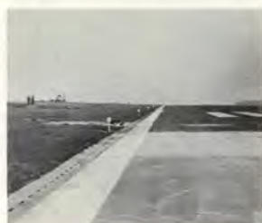
Blown tire from wheel striking barrier tape guide resulted in F-4 mishap. Compare photos above. Note edge striping, location of lights.
